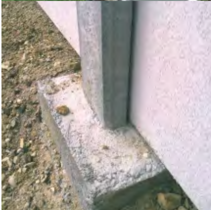
Fig. 6 First Course of Fence Panels.
