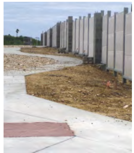
Fig. 8 Stepped Fence Layout.
