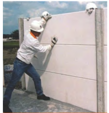
Fig. 7 Hebel® Fence Panel Installation.
