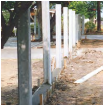
Cast in Place Base
