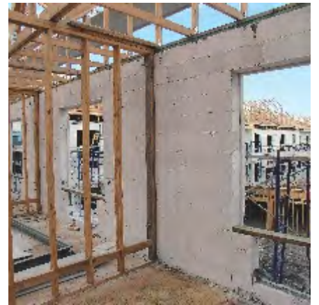
Fig. 21: Construction interior view.
