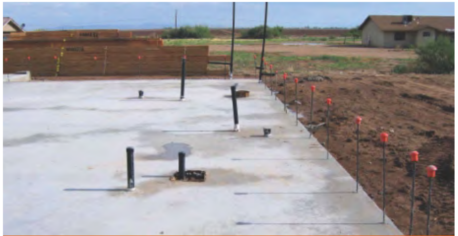
Fig. 6: Check foundation (pipes, drains, reinforcement, etc).
