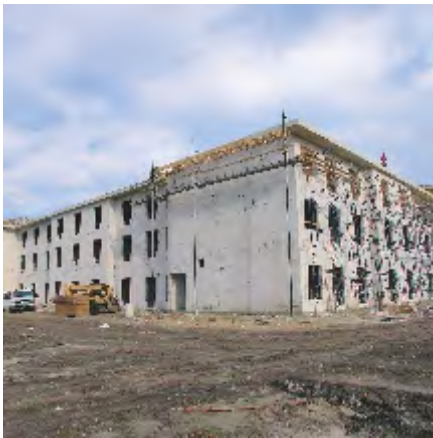
Fig. 22: Three-story hotel construction.
