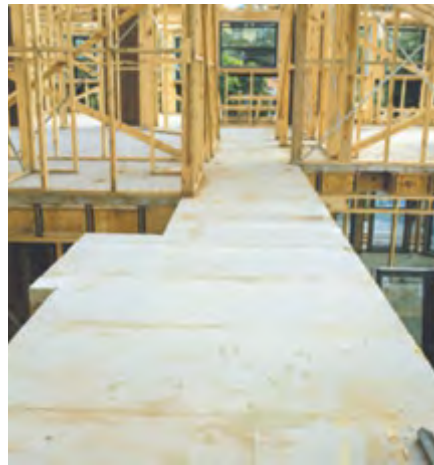
Fig. 7: Fitted Flooring with Internal Loadbearing Wall.
