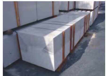
Fig. 5: Place Hebel® Power Floor™ pallets close to job site.
