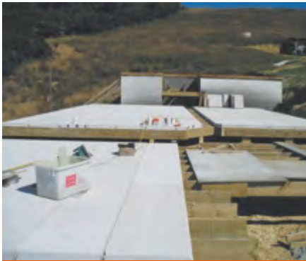
Fig. 10a : Hebel Power Floor at ground level.
