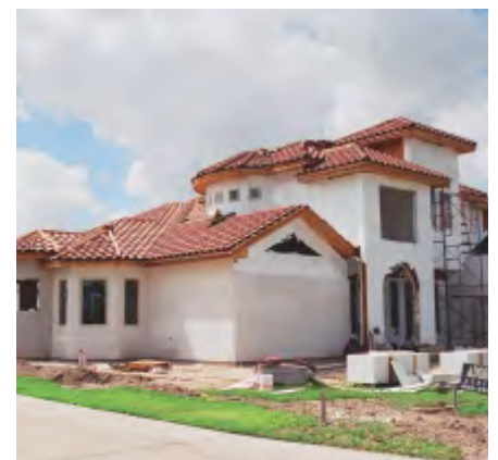
Fig. 4: Place Hebel® Power Panel pallets close to job site.
