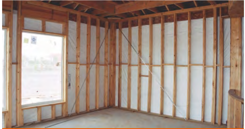
Fig. 5: Interior side of the water-resistant barrier.
