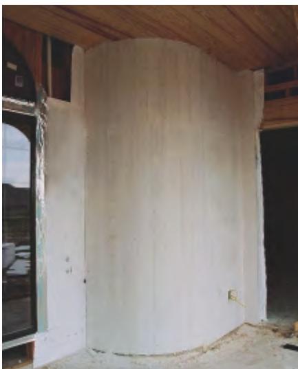
Fig. 13: Hebel® Power Panel circular wall.
