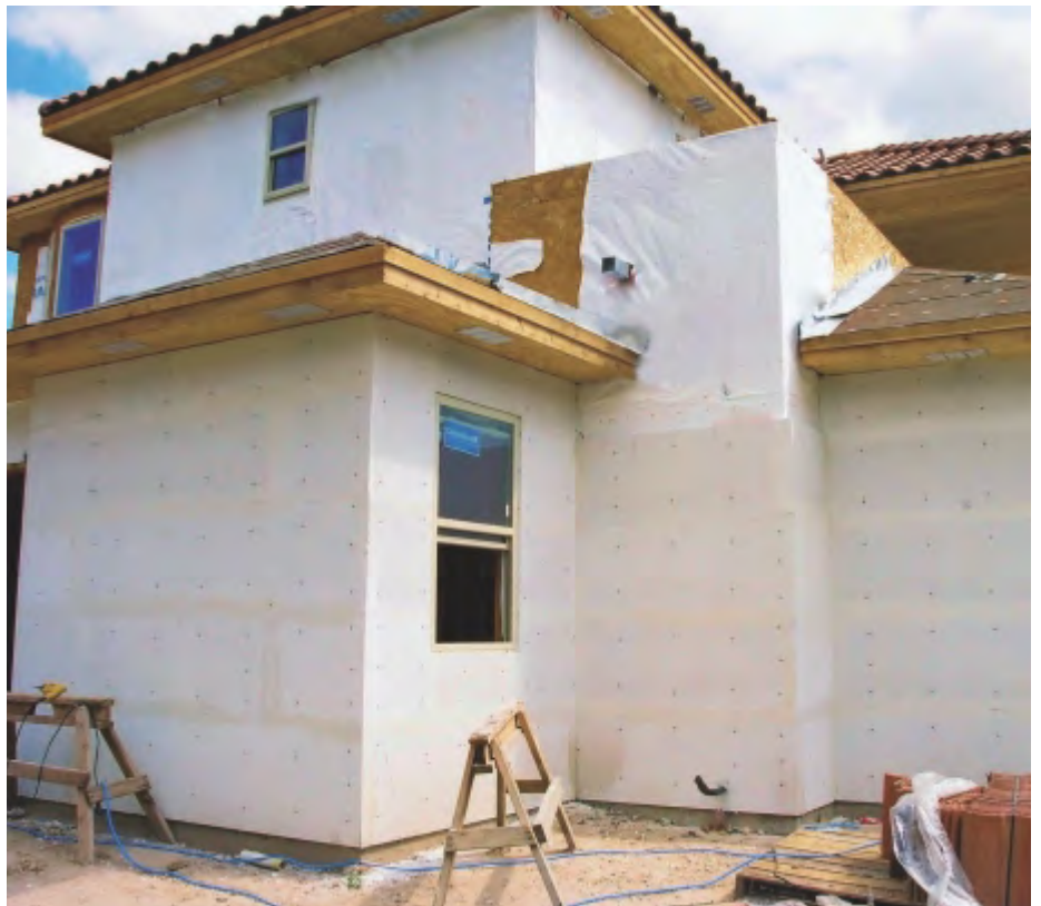
Fig. 15: Hebel® Power Panel on exterior walls.
