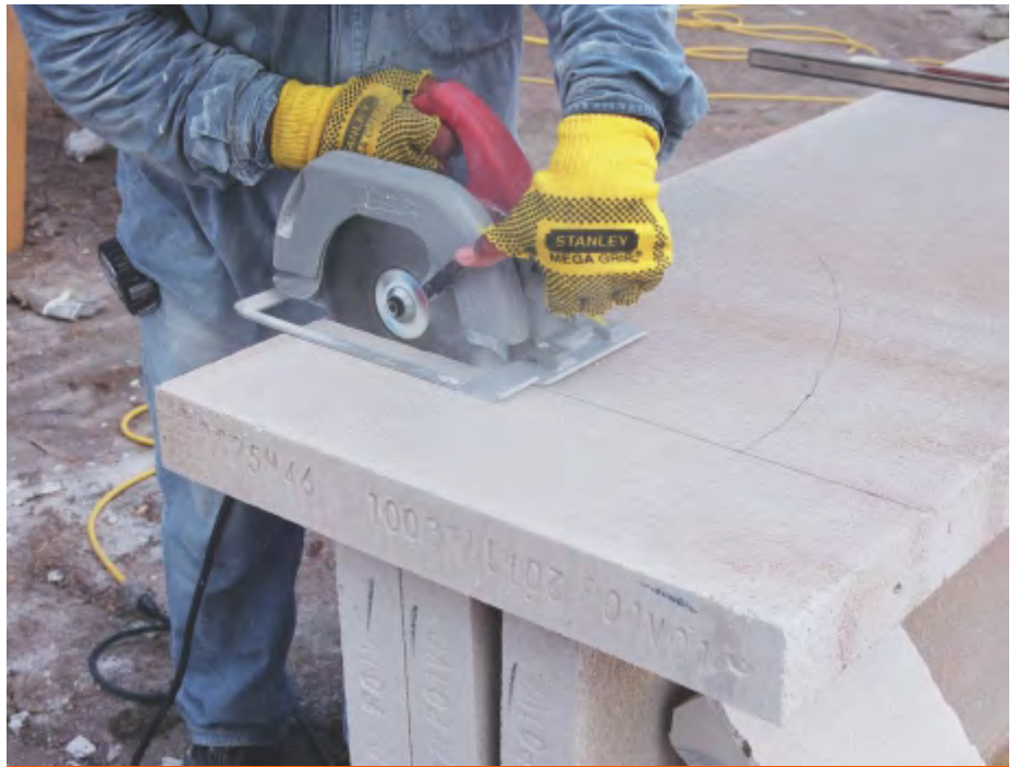
Fig. 14: Cutting Hebel® Power Panel using a circular saw.
