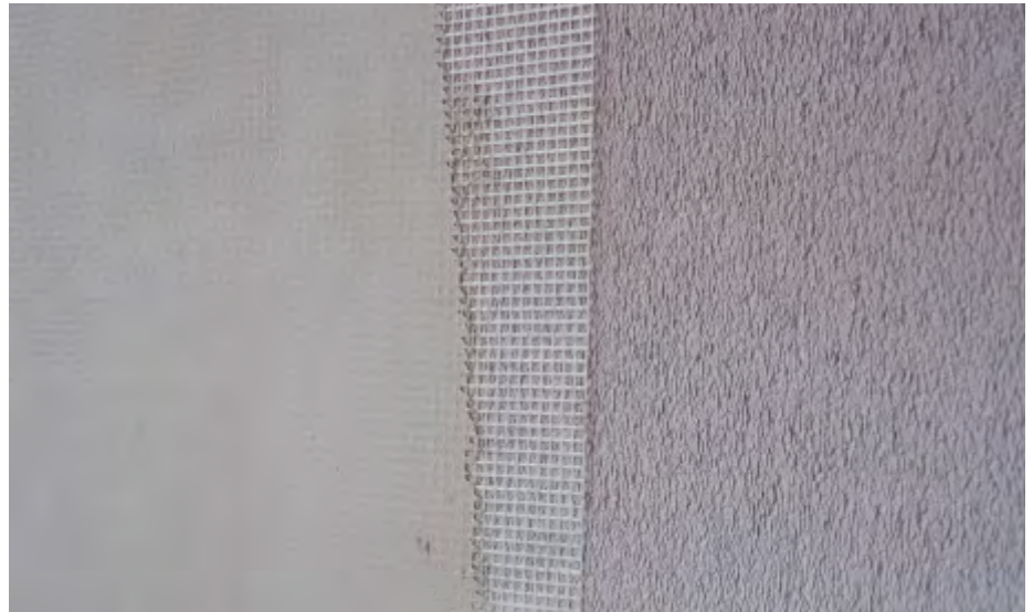
Fig. 17: Fiberglass mesh installation.
