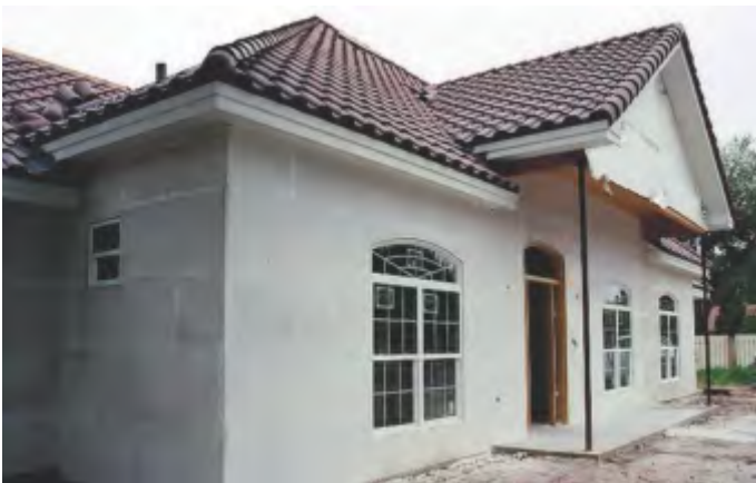
Fig. 12: Completed installation of an external wall using Hebel® Power Panel.
