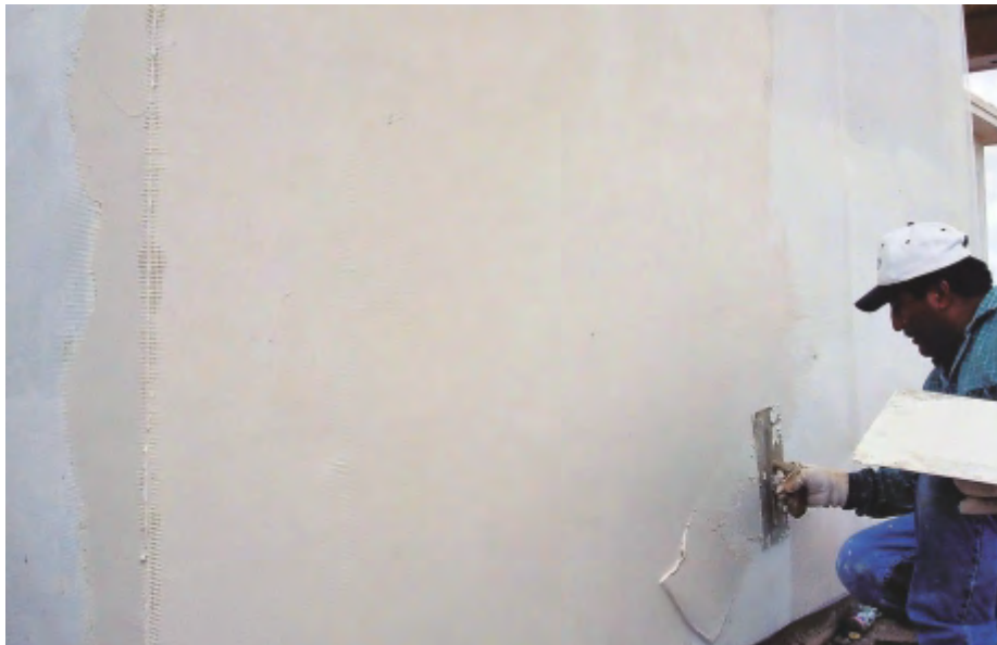
Fig. 16: Base-coat application.
