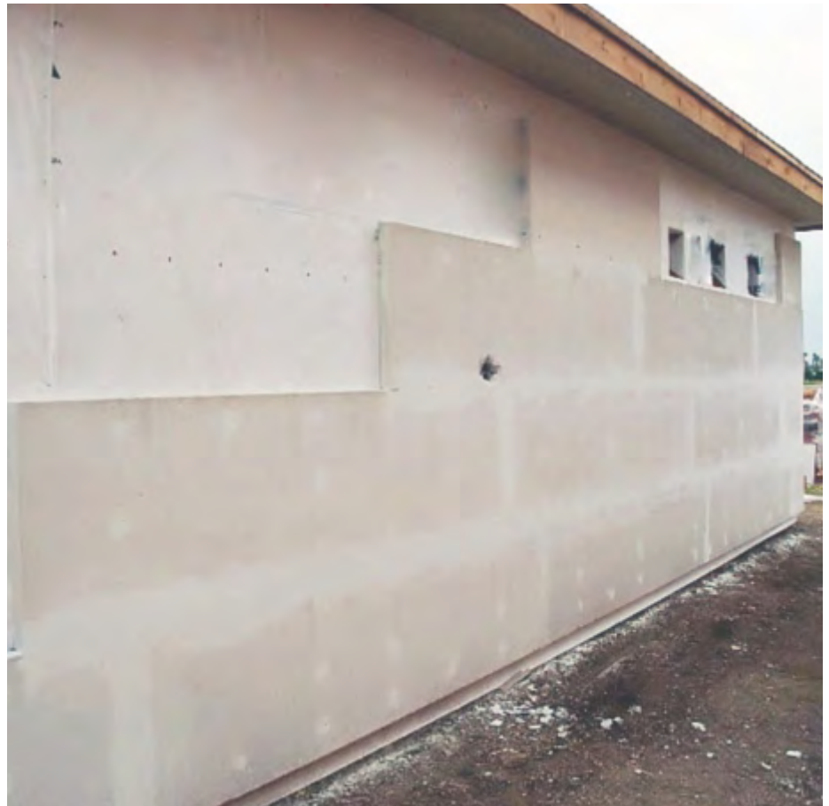
Fig. 9: Hebel® Power Panel in a running bond pattern.
