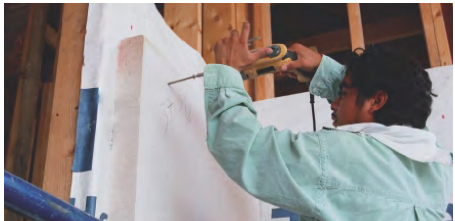
Fig. 7: Use minimum 3 fasteners per stud / board.
