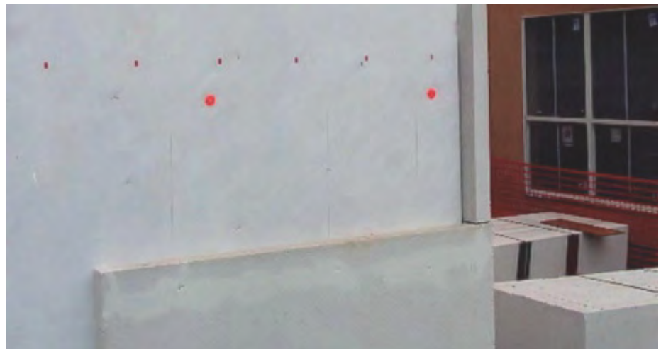
Fig. 6: Overlap Hebel® Power Panel at corners.
