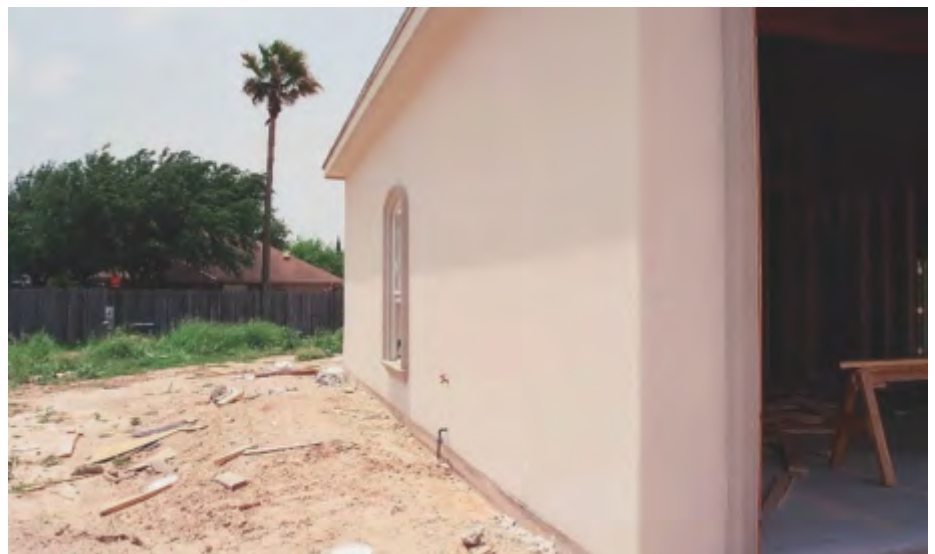
Fig. 18: Finished wall (base-coat and texture).
