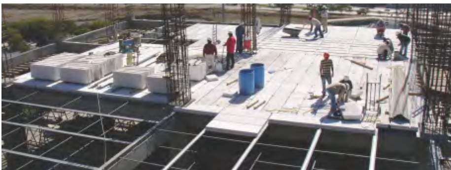
Fig. 5: Slab Panel supported by steel elements.
