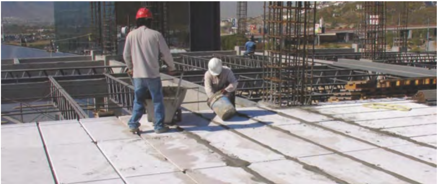
Fig. 18: Filling longitudinal joint with cement-sand mortar.
