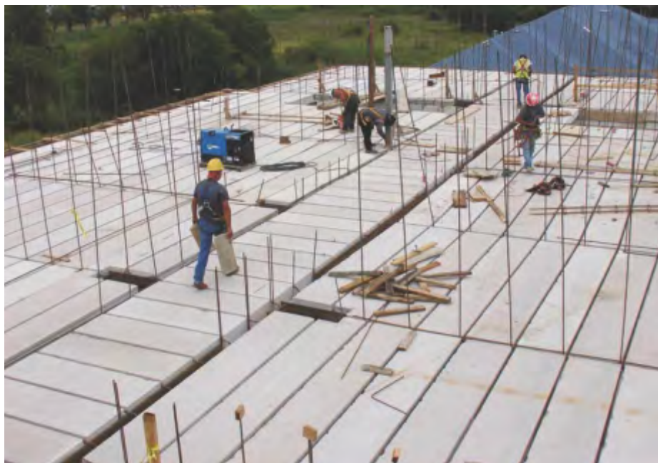
Fig. 15: Five-story hotel built with AAC (floor panels).
