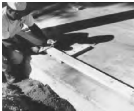
Fig. 10: Identify openings on template.
