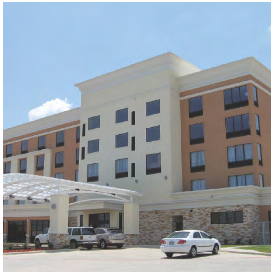
Fig. 27: Five-story hotel built with Hebel® AAC load bearing Wall Panels.
