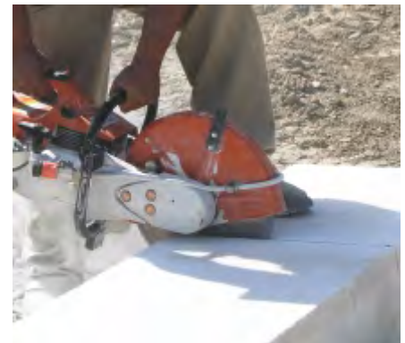
Fig. 25: Cut panels using a gasoline-powered circular saw.
