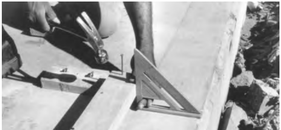
Fig. 9: Place template [elevated] on cleats to allow uniform distribution of mortar bed. Align template to building wall lines.
