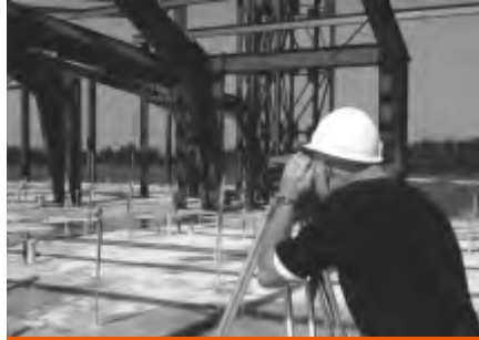
Fig. 6: Check the levelness of the slab prior to installing the template.
