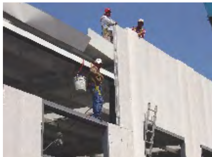
Fig.15: Plumbing the panel in second course.
