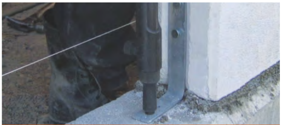
Fig.13: Fix the lower connector (type "B" connector).
