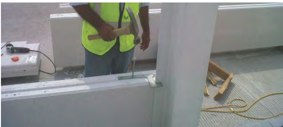
Fig.9: Nail the connector to the panel (type A connector).
