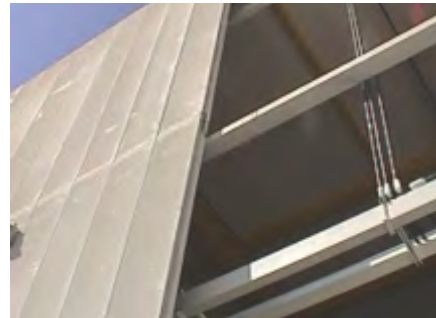
Fig.16: Second course of Hebel® Vertical Wall Panels.
