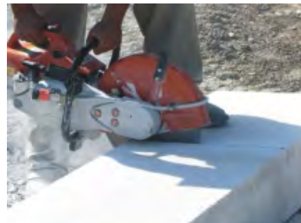
Fig.17: Cutting panel.
