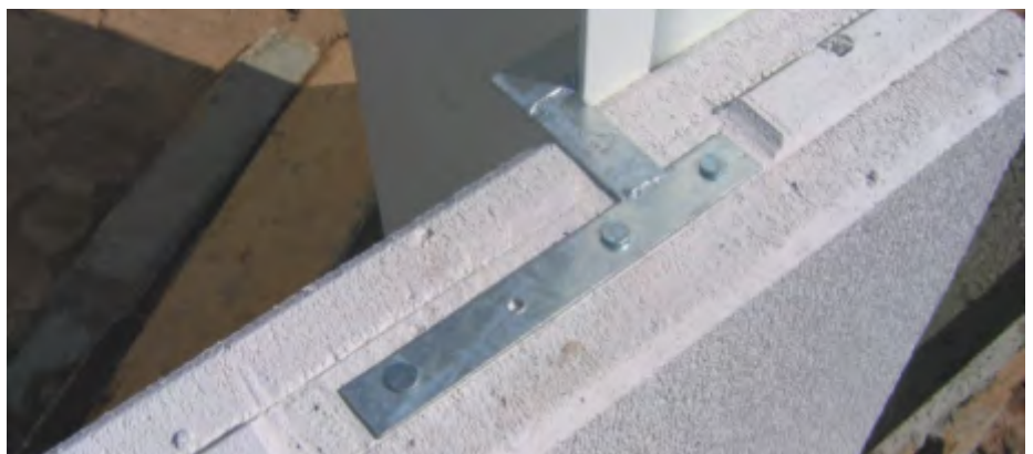
Fig.14: Typical upper connection (type "C" connector).
