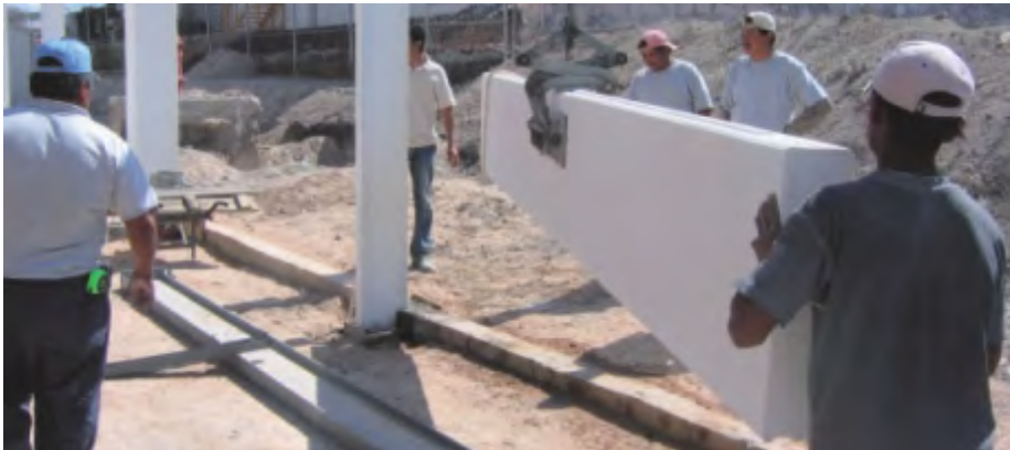
Fig.8: Place lifting gear at the center of the panel.
